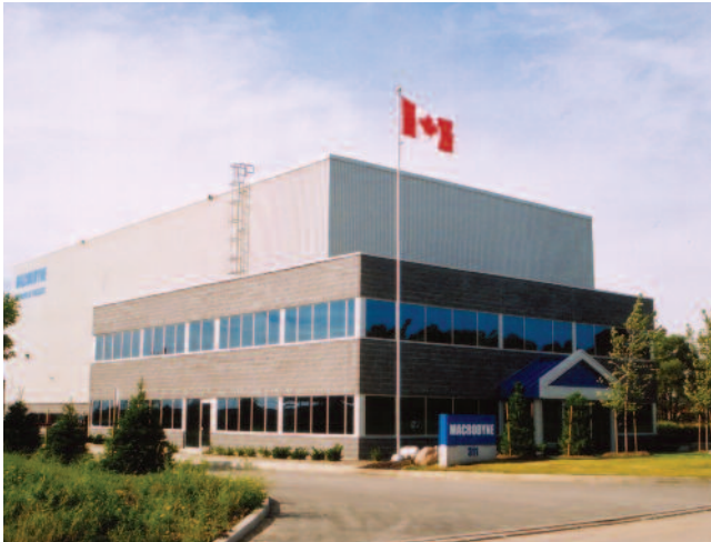
Custom designed hydraulic press factory
